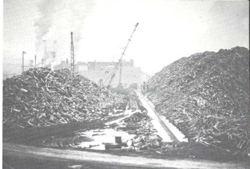
A half-hour's drive southeast of Andover is the Rumford-Mexico industrial complex. Dominating the industrial scene is the Boise Cascade paper mill, one of the largest of its kind in the world.
